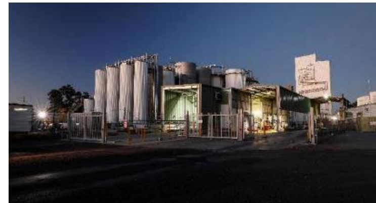
GrainCorp oilseed crush plant, Numurkah, VIC
