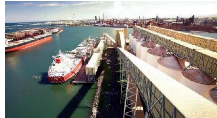
GrainCorp bulk port terminal, Port Kembla, NSW
