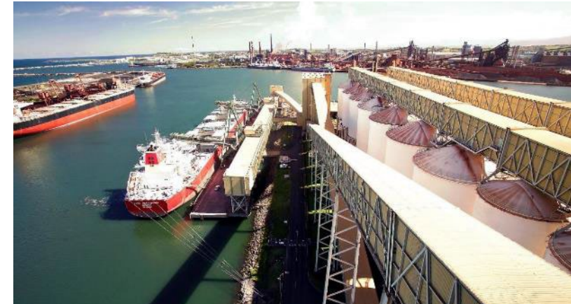
GrainCorp bulk port terminal, Port Kembla, NSW
