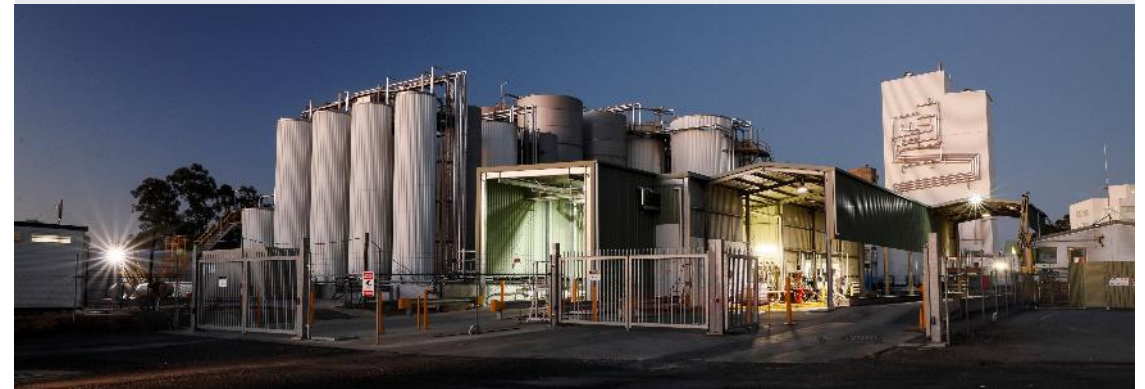
GrainCorp oilseed crush plant, Numurkah, Victoria
